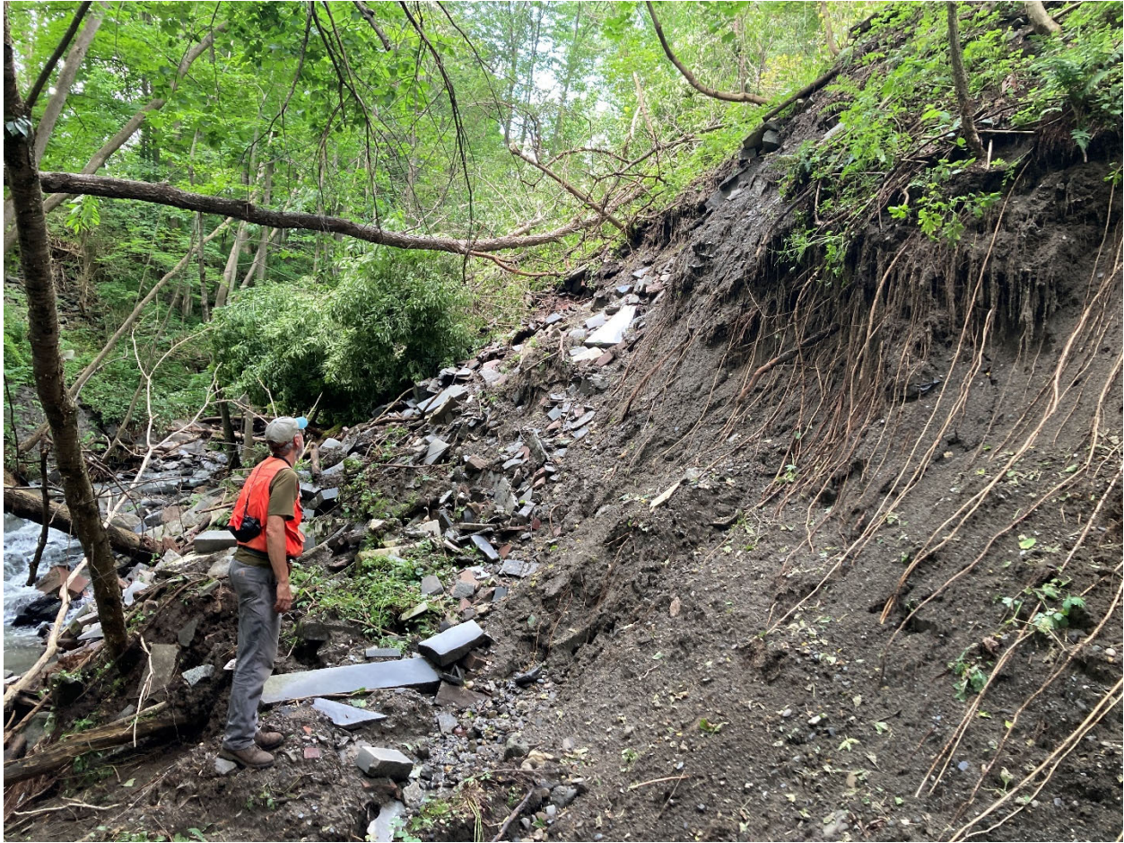
Photograph 4: Same view as Photograph 3 looking north with a close-up view of fill materials making up the slope below 106 Currier Street. Note the roots hanging over the edge of the slope that were exposed following failure of the slope base, as well as fallen trees in the background; geologist for scale.
