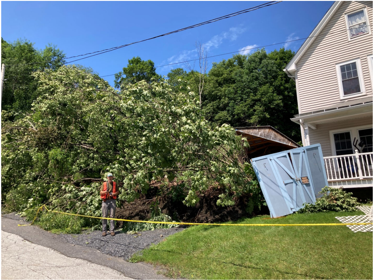
Photograph 2: The toe of the landslide at 25 Oswald Street on July 14, 2023. The farthest traveled landslide debris came to rest against the exterior wall of the house at 19 Oswald Street shown on the right in this picture; geologist for scale.
