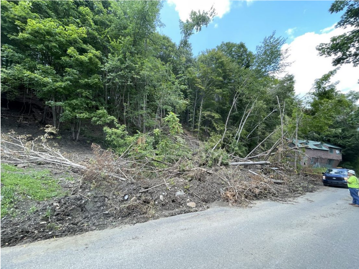
Photograph 4: View of the house and landslide debris along Portland Street. Photograph taken August 4, 2023.
