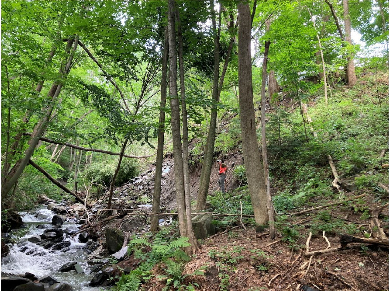
Photograph 3: View looking north along the brook at the base of the slope below 106 Currier showing the failed base of the slope. The residential structure at 106 Currier Street is located directly on top of this slope; geologist for scale.
