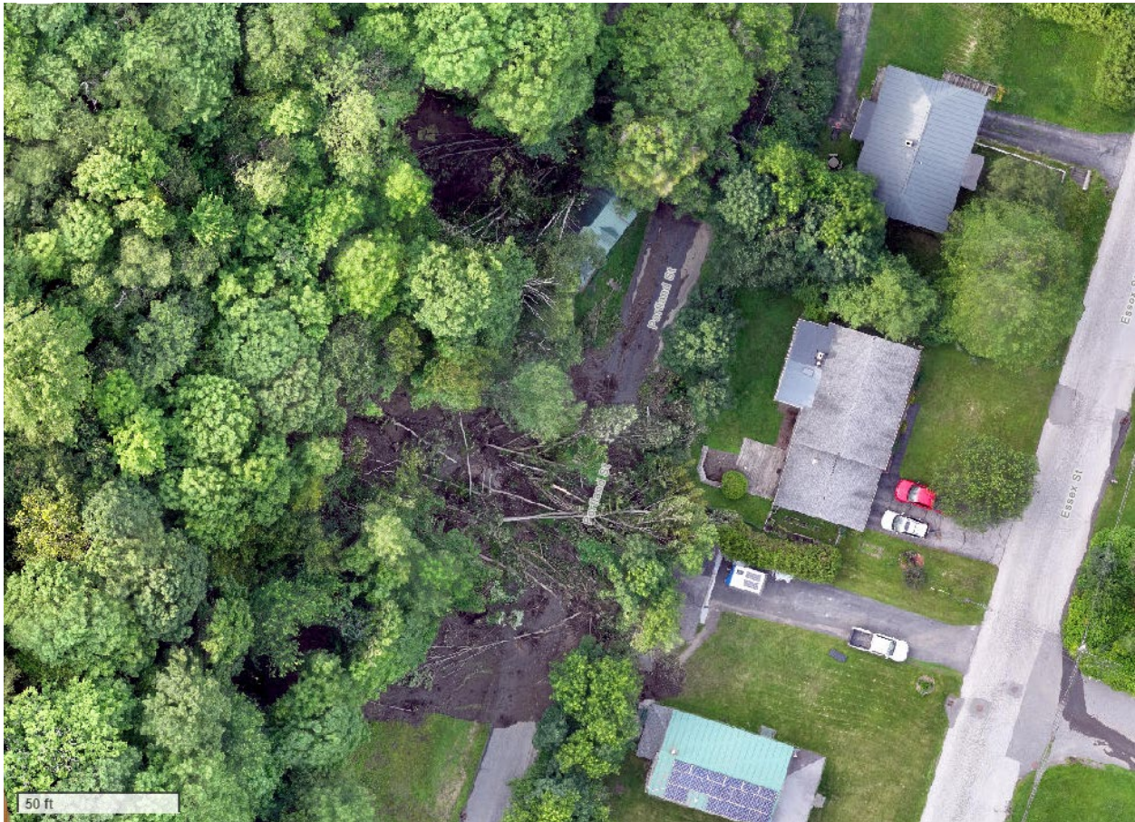
Photograph 2: Aerial drone imagery taken on July 12, 2023 showing the failed slope and landslide debris prior to cleanup along Portland Street. The destroyed house at 5 Portland Street is visible in the upper center of the photo. Note the additional large landslide debris lobe into Portland Street further to the south.
